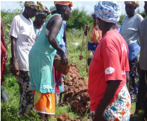
Photo 5: Women building an anti-erosion ring
